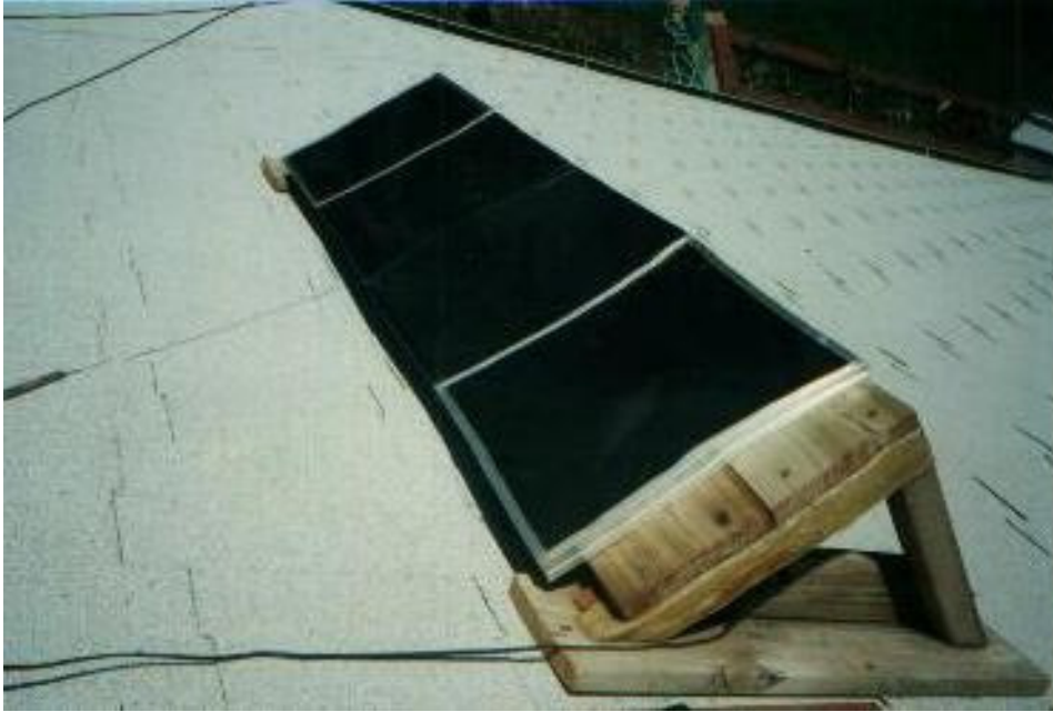
Solar panel on the roof
